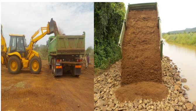
Ferrying of stones and gravels for the road work
