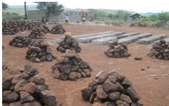
Local materials (Sand and stones) collected for construction of the secondary school classroom
