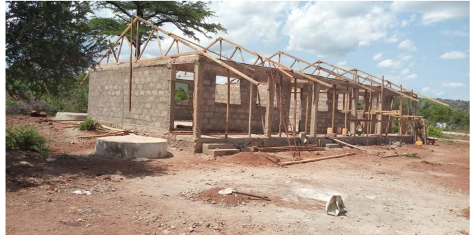
Roofing of the secondary school classrooms
