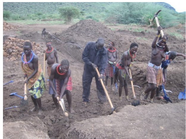
Construction of an Irish bridge near the air strip
