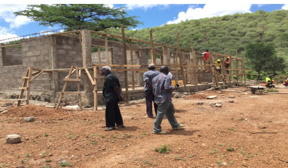
Construction of the secondary school classroom.
