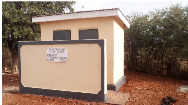
Latrine with two stances constructed by VTS for the ECC centre at Lorusothuko
