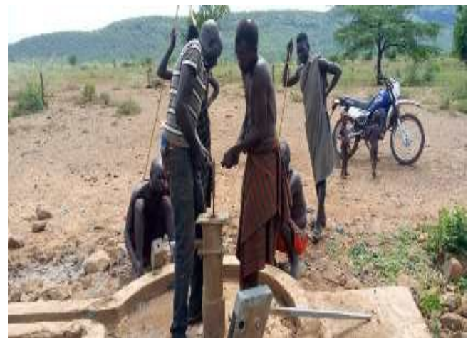
Repair of damaged bore holes in the villages around HTPVK
